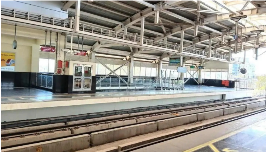
Nagpur railway station ??????????
