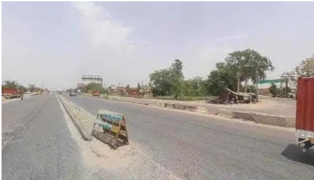
Hsiidc ie dharuhera site office ellaam
